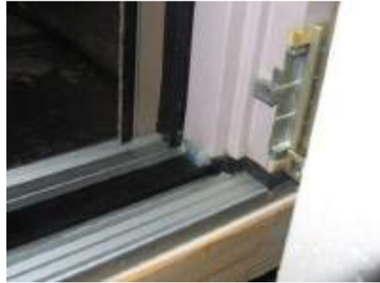
Photo 8 Centre seal, sealant joint
