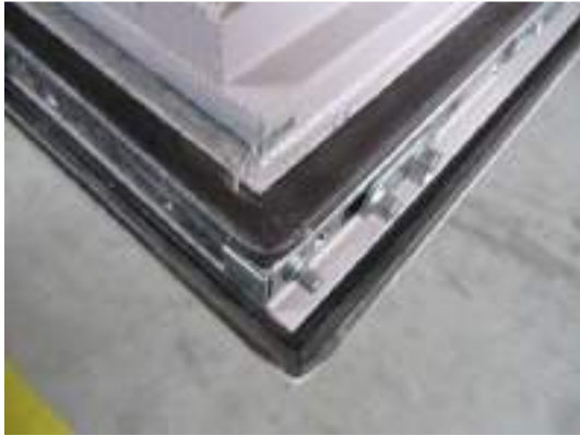
Photo 13 Sash seal, corner configuration
