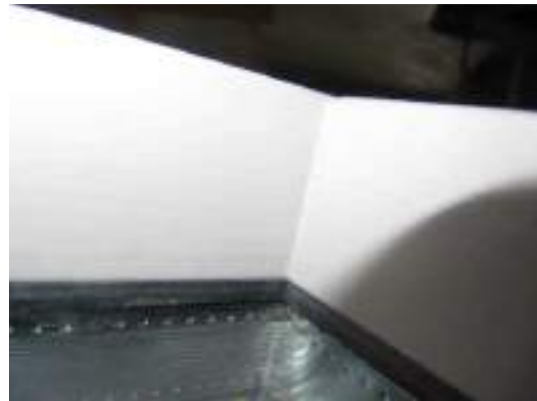
Photo 22 Internal glazing seal, corner configuration
