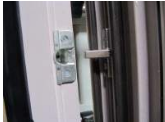
Photo 30 Locking situation, frame / sash, rear-engaging
