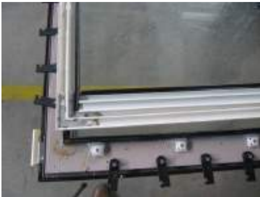
Photo 21 External glazing seal, sealant joint
