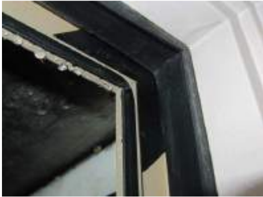
Photo 7 Centre seal, corner configuration
