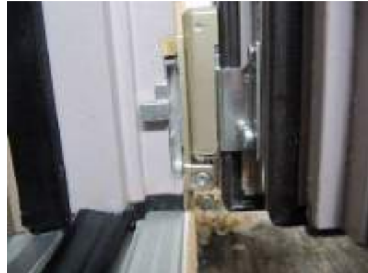
Photo 28 Corner pivot, rebate view
