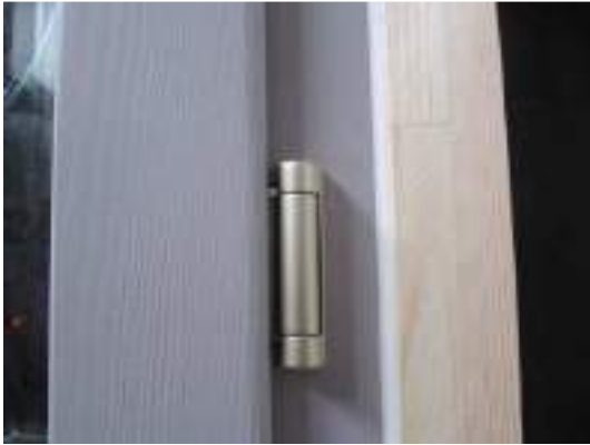
Photo 25 Turn mechanism pivot, internal view
