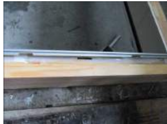
Photo 4 Rebate drainage to outside
