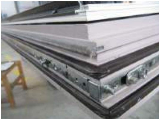
Photo 9 Centre seal on sash, brush gasket, corner configuration,
