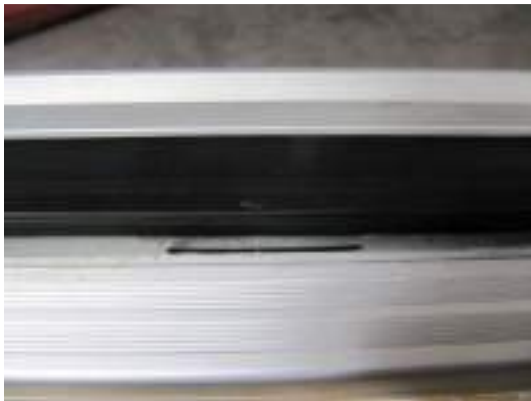
Photo 3 Rebate drainage on threshold
