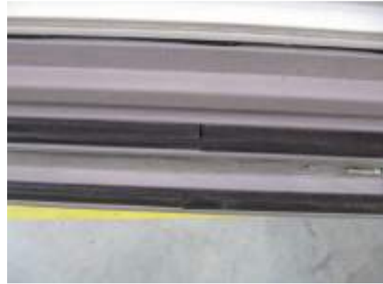
Photo 14 Sash seal, sealant joint
