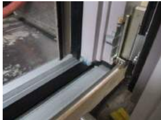
Photo 10 Threshold seal, sealant joint
