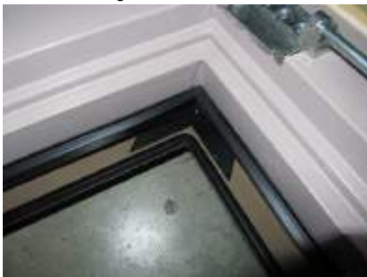
Photo 5 External rebate seal, corner configuration
