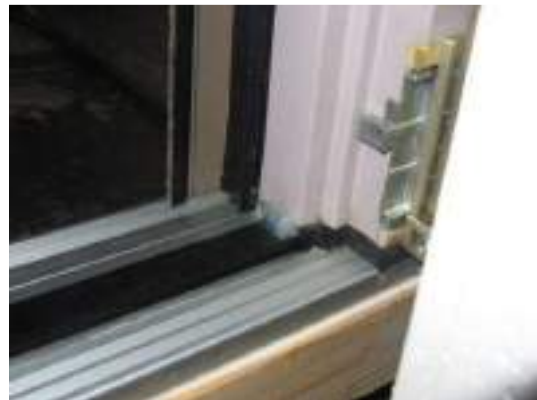
Photo 12 Threshold seal, additional sealed with pourable sealant lateral
