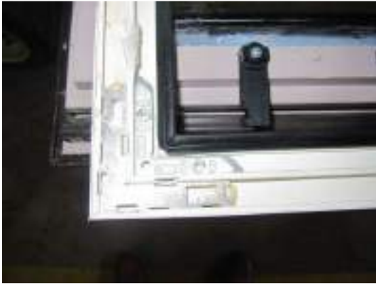
Photo 19 External glazing seal, corner configuration
