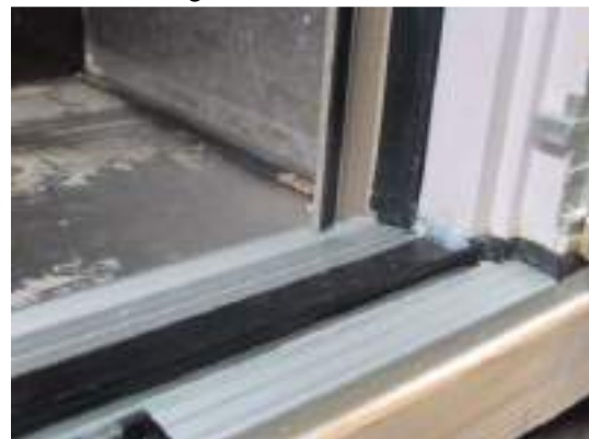
Photo 6 External rebate seal, sealant joint
