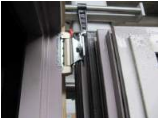
Photo 29 Turn mechanism pivot, rebate view, at top
