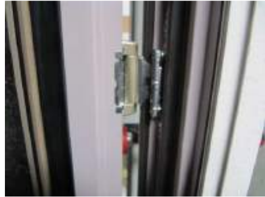
Photo 26 Turn mechanism pivot, rebate view
