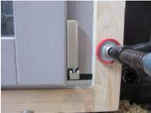
Photo 27 Corner pivot, internal view
