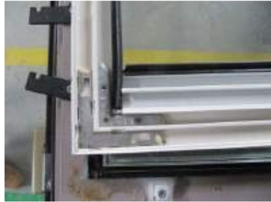
Photo 20 External glazing seal, sealant joint
