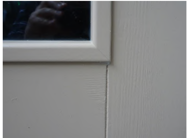
Picture 16 Internal glazing bead and glazing corner
