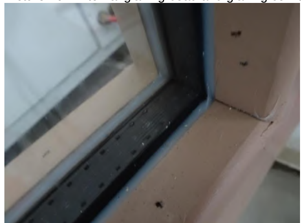
Picture 18 Sealing of glazing, seen from outside
