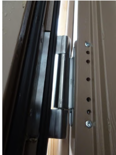
Picture 8 Hinge seen from rebate, at bottom
