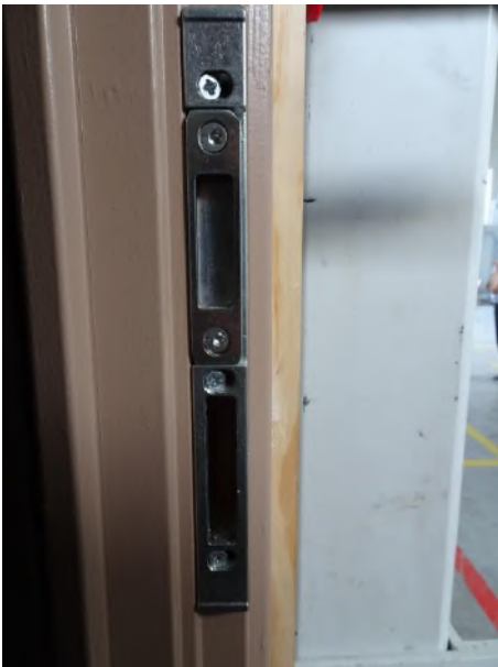
Picture 21 Strike plate for main lock
