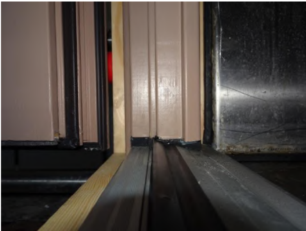
Picture 13 Threshold, seen from rebate
