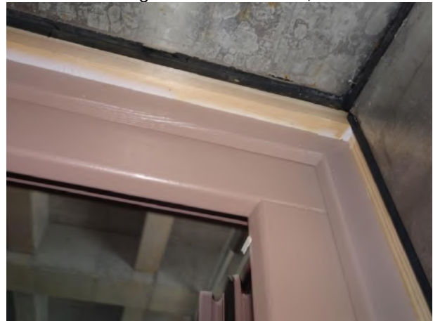
Picture 10 Frame at top, corner design, seen from outside
