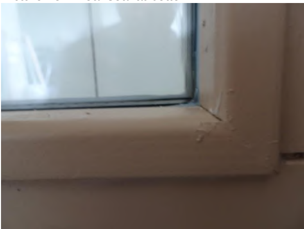
Picture 17 External glazing bead and glazing corner
