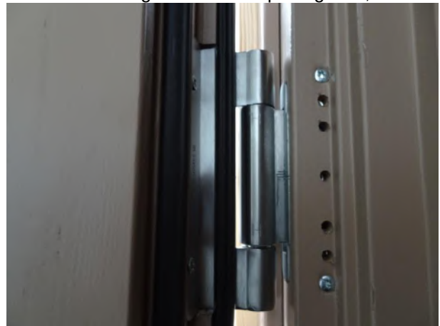
Picture 6 Hinge seen from rebate, at top
