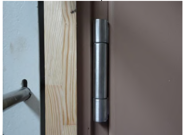
Picture 4 Hinge seen from opening side, at centre
