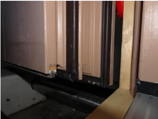
Picture 15 Leaf seal at bottom
