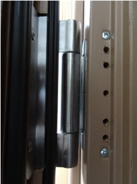
Picture 7 Hinge seen from rebate, at centre
