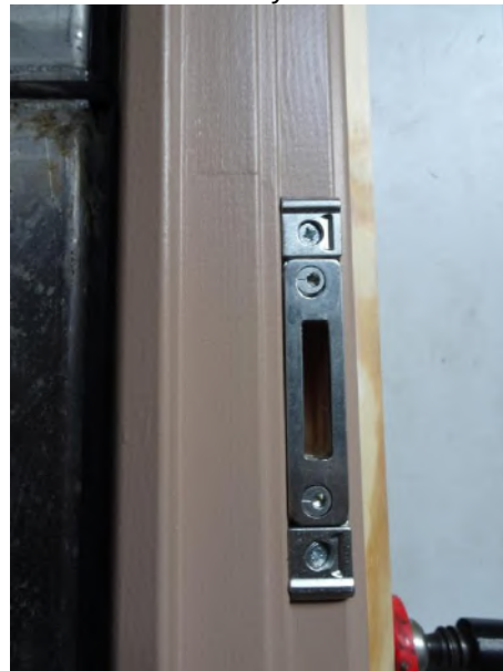
Picture 22 Strike plate for auxiliary lock
