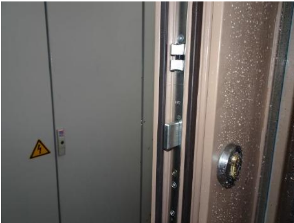
Picture 19 Main lock
